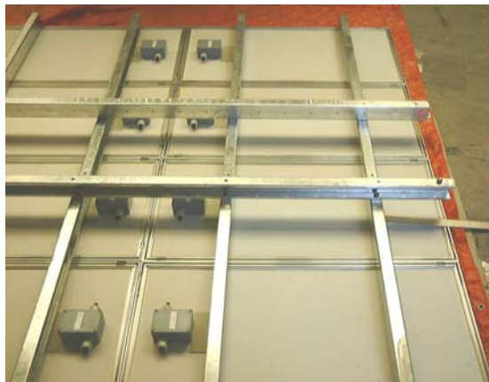
The solar module beams are connected to the traverse beams
